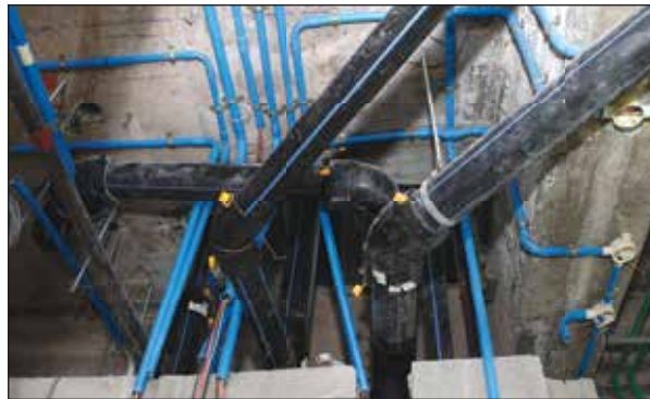
RFL HDPE Sewerage Pipe Line at Hotel Intercontinental, Dhaka
