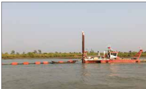
RFL HDPE Dredging Line at Cox's Bazar air port extension work
