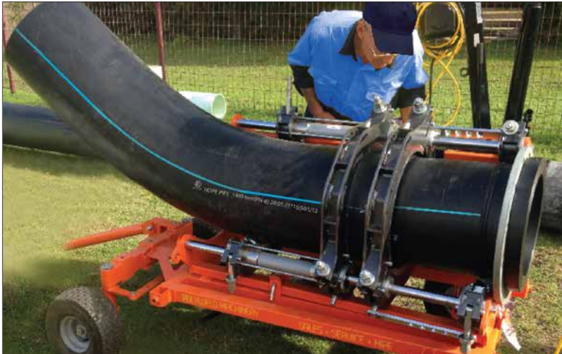
Butt Fusion Welding
