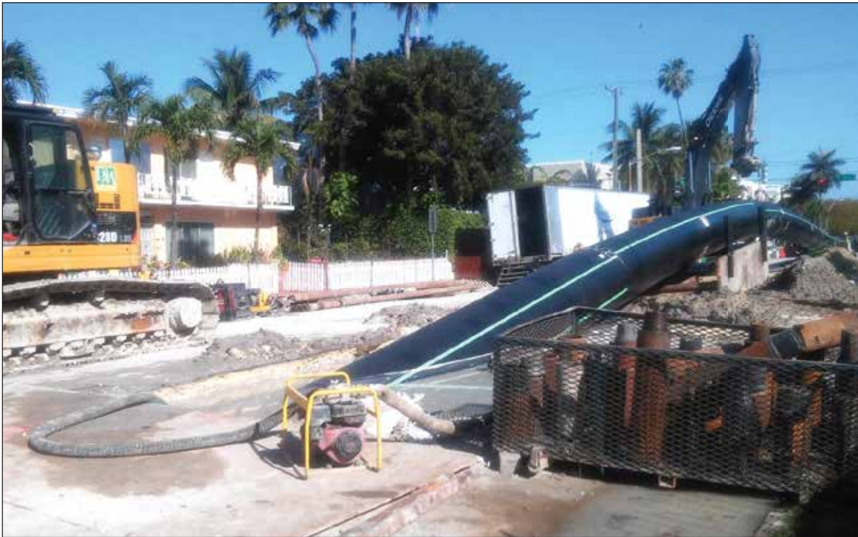
RFL HDPE Pipe Laying
